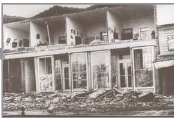
1906—Damage in Healdsburg
