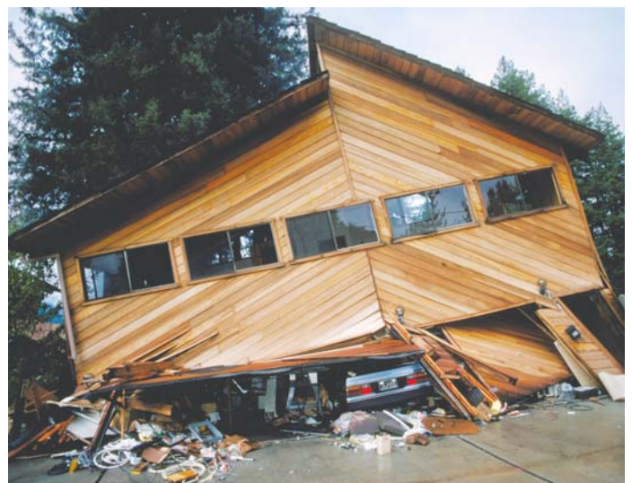
This home in the Santa Cruz Mountains, California, collapsed in the 1989 magnitude 6.9 Loma Prieta earthquake (USGS photo).
