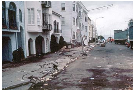
Liquefaction —Earthquake shaking can cause soils to behave like a liquid and lose their ability to support structures. Liquefaction often causes buried gas and water lines to break. The highest hazard is in low-lying areas where there are loose, sandy soils or poorly compacted artificial fill. This photo shows liquefaction-related damage in the Marina District of San Francisco following the 1989 magnitude 6.9 Loma Prieta earthquake (USGS photo).
