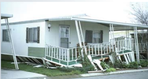
Mobile home damage in the 1980 magnitude 5.8 Livermore earthquake (photo courtesy NISEE).
