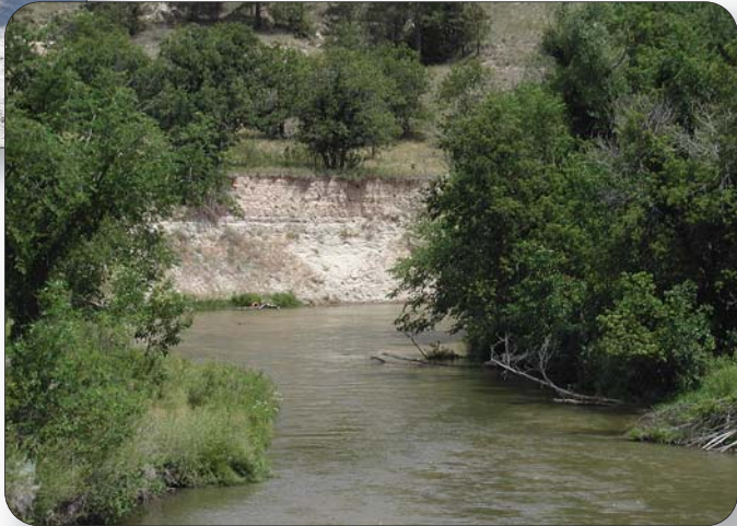
Streambank available for collapse and movement downstream during higher flows.
