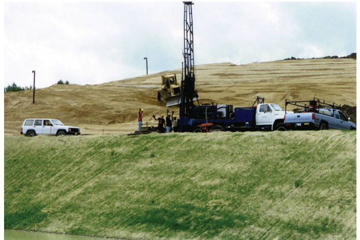
Photo 1. Drill rig installing monitor well at Saco Area 4 Landfill (landfill forms hill in background).
