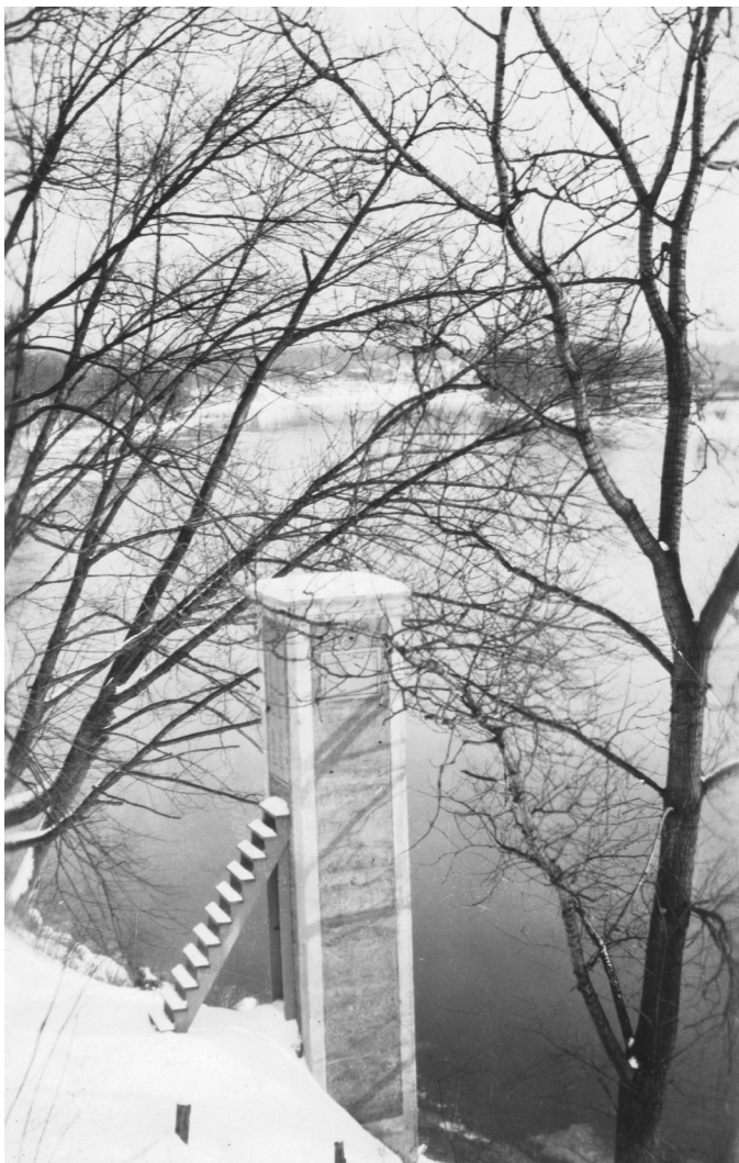
Figure 2. The Montague City, Massachusetts, streamflow-gaging station, shortly after its construction in October 1929.
