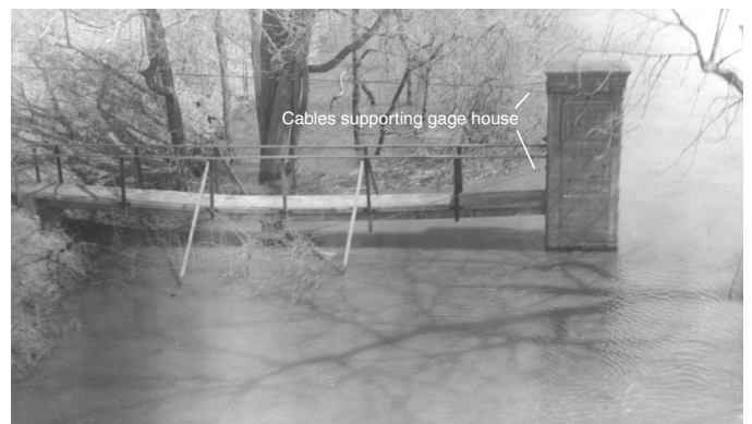
Figure 4. The Montague City station under high water, April 6, 1960. Recorded stage was 37.50 feet.
