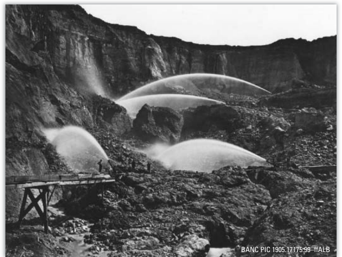
Figure 4. The Gold Rush of the 19th century caused a population explosion in California and led to the first major manmade changes to the region’s landscape. This photograph shows high-pressure water cannons (monitors) washing down gold-bearing gravel at the Malakoff Diggings in the foothills of the Sierra Nevada. Such destructive hydraulic mining methods, later outlawed in California, sent enormous quantities of sediment down the rivers and into San Francisco Bay, where it reduced the water depth over large areas. (Photograph by Carleton E. Watkins, courtesy of the Bancroft Library, University of California, Berkeley.)
