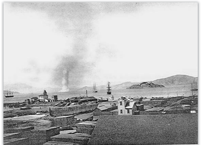
Figure 7. Blasting of Arch Rock in 1901 is seen in this photograph taken from San Francisco. Alcatraz Island is in the right middle ground. (Photograph courtesy of U.S. Army Corps of Engineers.)
